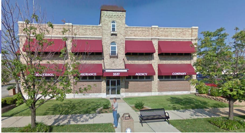
3537 South Kingshighway - Before
