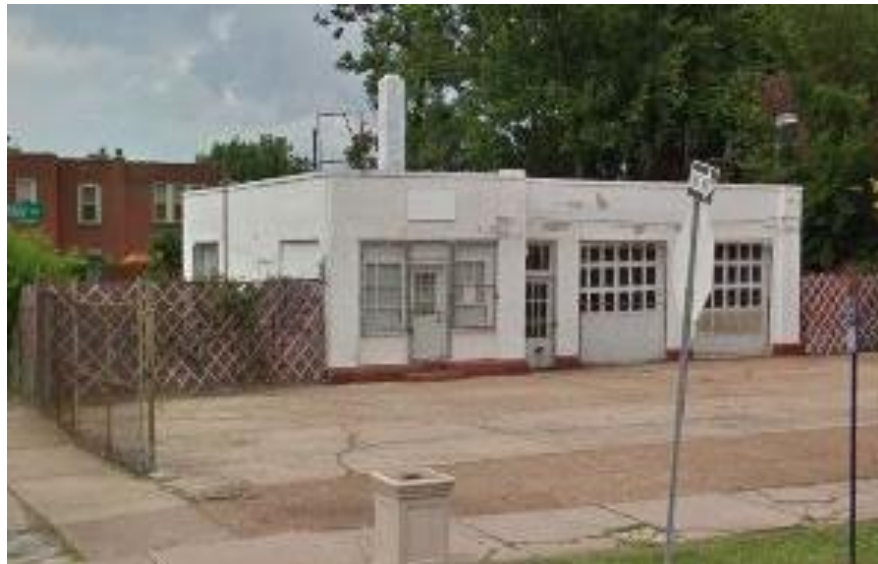
4175 Shaw former Gas Station
